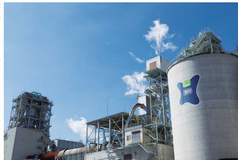
Eco-Cement plant, which produces cement from incinerator ash
