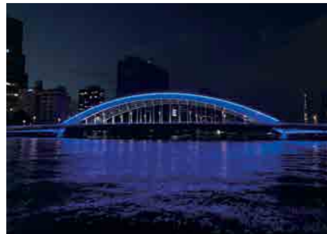
Rebuilt in 1926 after the Great Kanto Earthquake, Eitai Bridge has been equipped with bearings to dampen large seismic forces.
