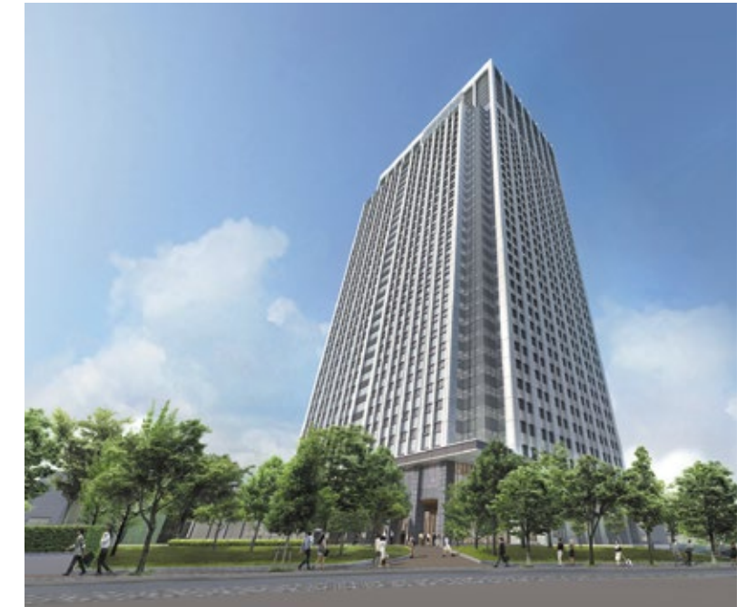
Tokyo World Gate opening in spring 2020 will have a 3,000-square-meter pedestrian green corridor including a stream.
