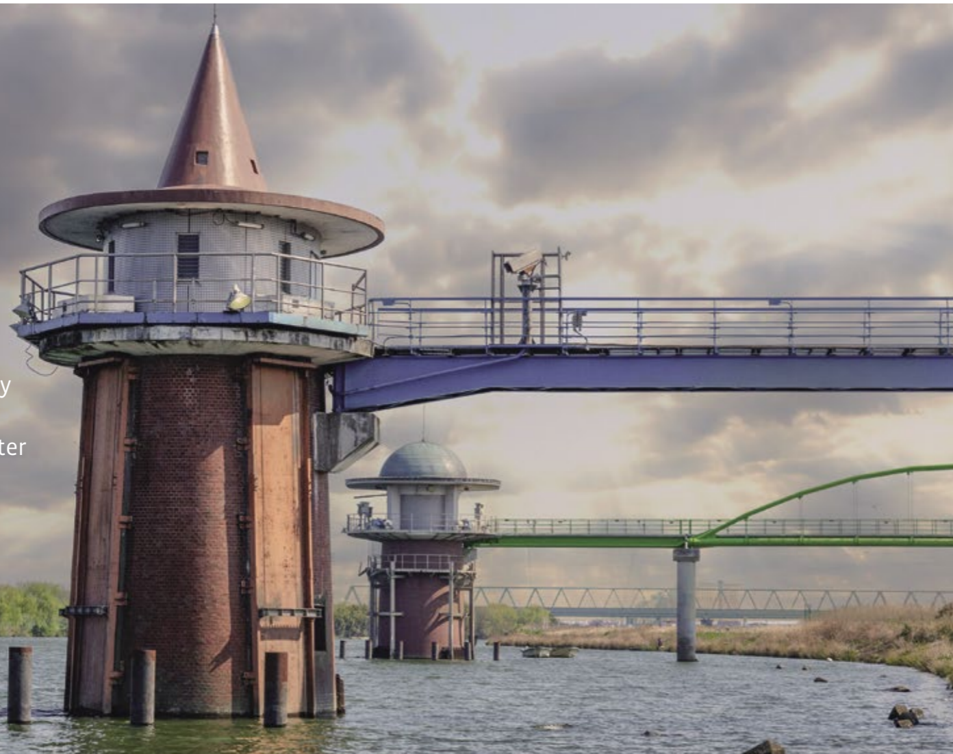
The iconic red brick intake tower of the Kanamachi Purification Plant, on Tokyo's Edogawa River.
