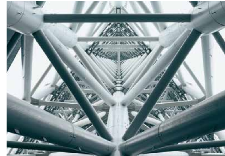
The truss structure of TOKYO SKYTREE is made of steel components that are approximately twice the highest value, as strong as those used in standard steel frames.
