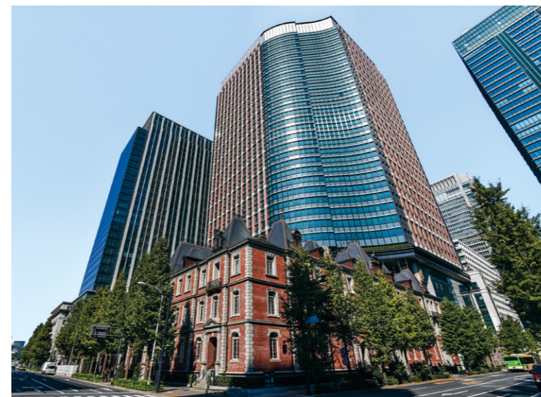
The Mitsubishi Ichigokan Museum, a reconstruction of the original Ichigokan, completed in 2010. Photo: iStock
