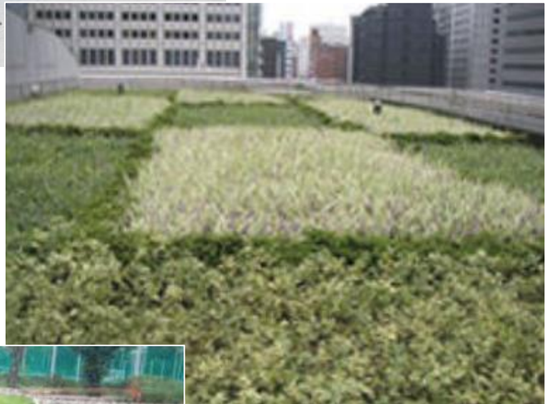
Rooftop greening (On the roof of the Tokyo Metropolitan Assembly building)
