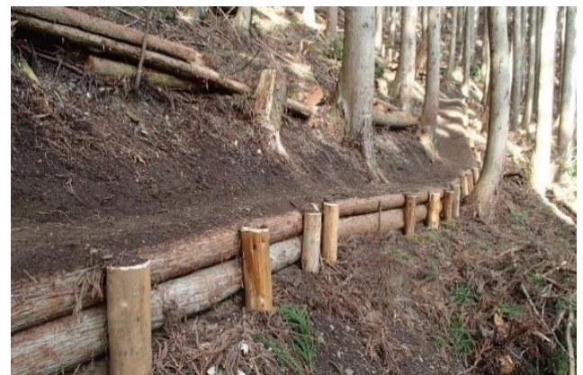
Maintaining a path for forest management (fence made from timber from thinning)
